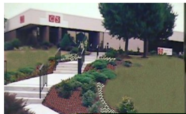
CTS USA Facility, Audobon, PA
